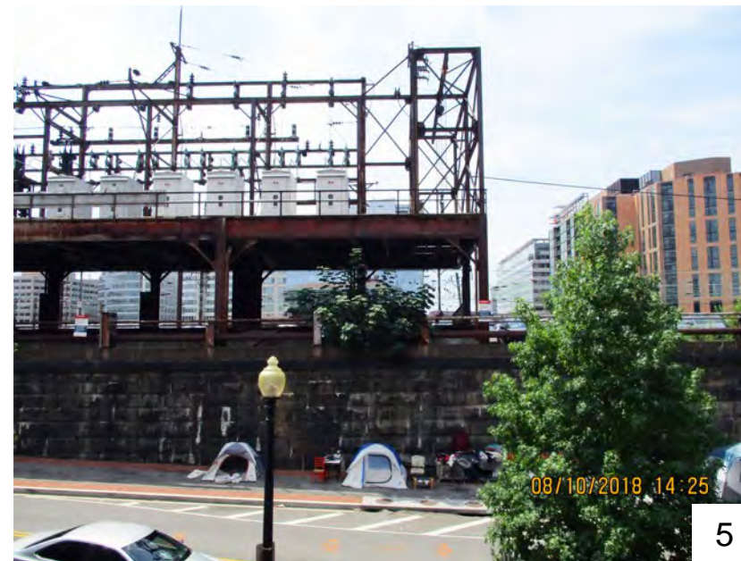
5 looking west from site at retaining wall & train tracks
