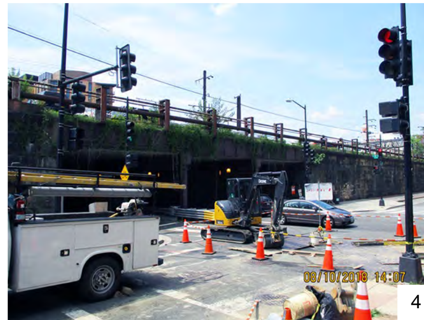
4 looking northwest at K St. underpass from 2nd & K NE intersection
